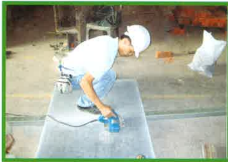
4 Cutting of ConcritBoard using electric cutting tool
