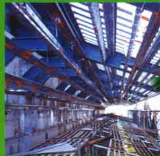
False Ceiling Construction
