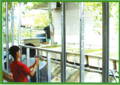
1 Fixing of steel studs
