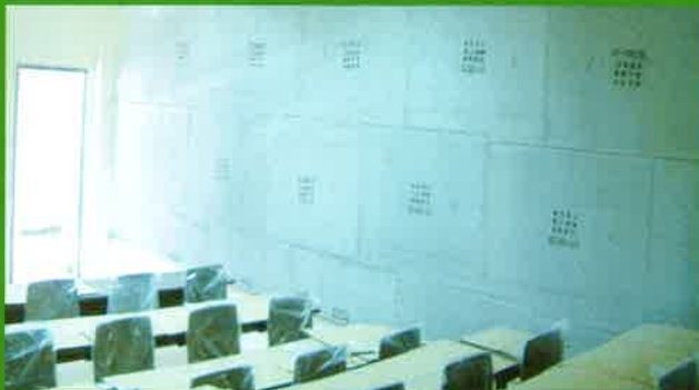
Taiwan - Training Center Wall Partition (Sound Acoustic Value STC 51)
