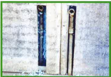
1 ConcritBoard can be easily cut on site to conceal services and pipes
