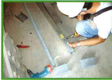
2 Cutting of steel stud using simple cutting tool
