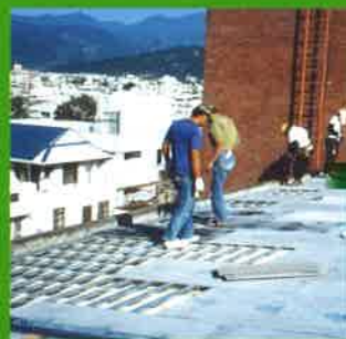
New Roof Construction
