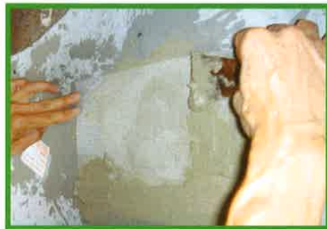
4 Overlay new fibremesh
