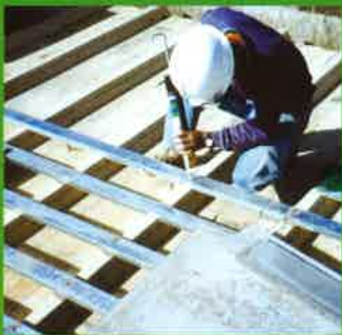
New Floor Construction
