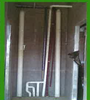
Singapore - Bathroom Wall Partition
