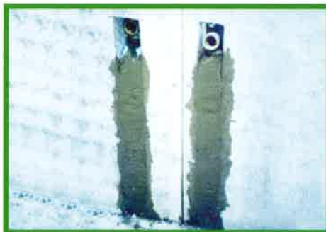
2 Cut-outs can be easily patched back by using cement + sand + water mixture
