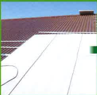
Taiwan - Overlay ConcritBoard on Existing Zinc Roof
