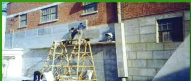
China - ConcritBoard Clad onto Brickwall
