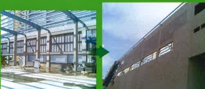
Singapore - Factory Façade Wall (Replace Aluminium Cladding Façade)
