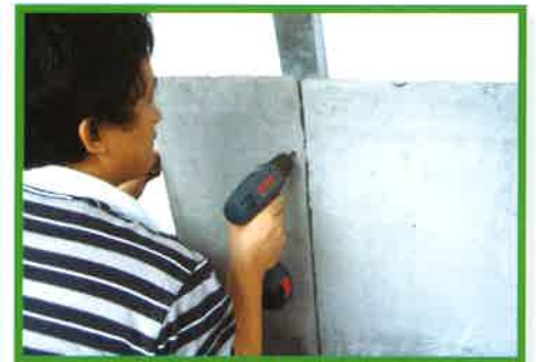
6 Fixing of ConcritBoard onto steel stud using battery drill & self-drilling screws
