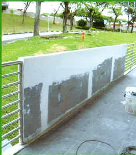
Singapore - Parapet Wall
