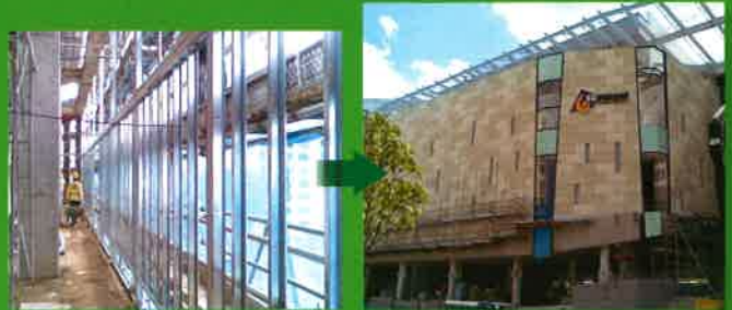
Singapore - Woodlands Church Façade Wall
