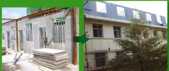
China - Lan Zhou Hospital – 3rd Floor Extension
