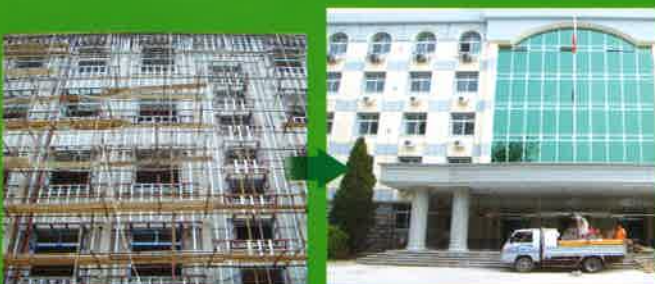
China - ConcritBoard Overlay on Old Façade Wall (School Project)
