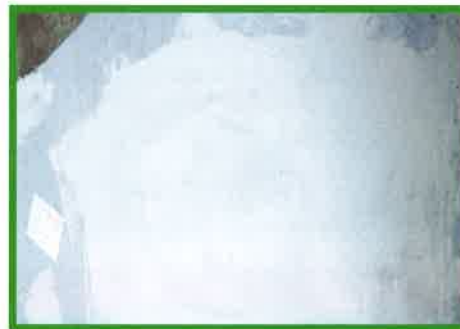
5 Skim coat the surface to smoothen it
