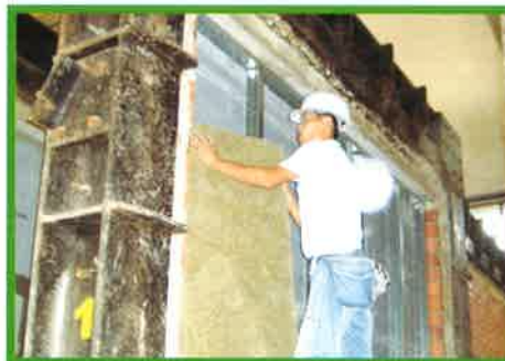
8 Install RockWool (if requiring acoustic & fire rating properties)
