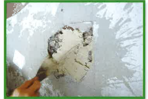
3 Patch dented area with cement + sand + water mixture
