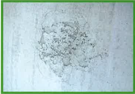
1 Damaged ConcritBoard caused by strong impact
