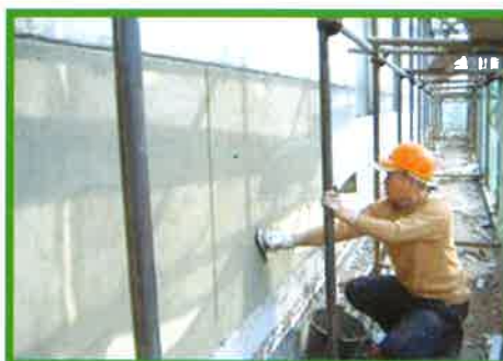
11 Smoothing the surface using recommended skim coat material
