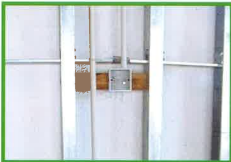
7 Running electrical services inside wall partition
