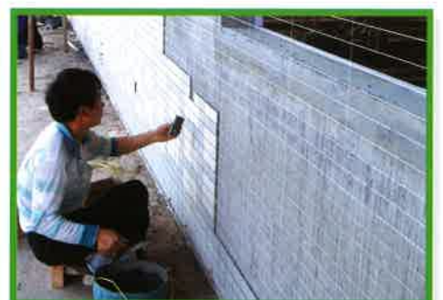
OR Laying tiles on ConcritBoard using normal tile adhesive (Fibremesh and skim coat can be obseleted for wall-tiled surface)
