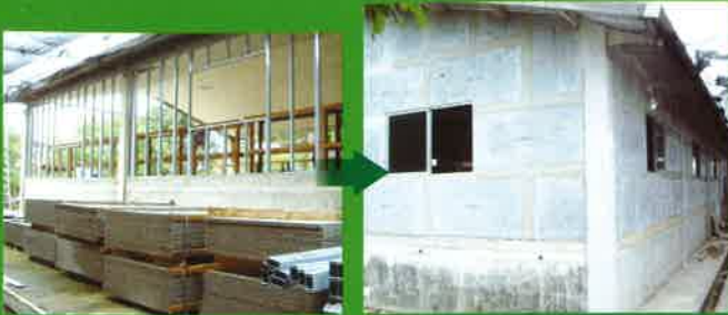
Singapore - Crab Farm Warehouse Construction
