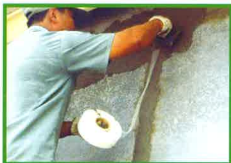
10 Reinforcing joints with a layer of fibremesh
