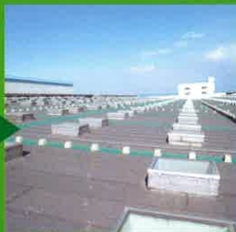
Taiwan - Overlay ConcritBoard on Existing Zinc Roof
