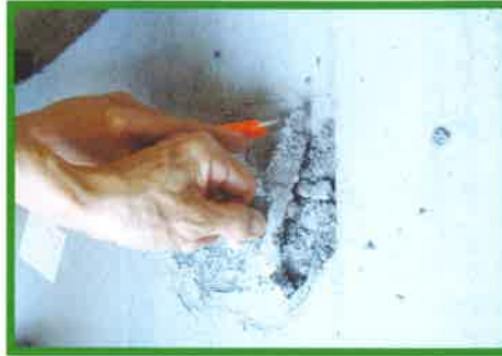
2 Cut and remove fibremesh
