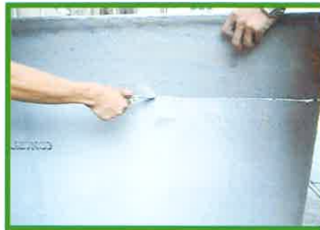
5 Alternatively cutting ConcritBoard using pen-knife
