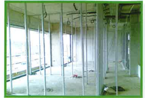
3 Completed steel stud frame
