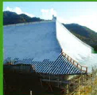
Taiwan - Temple Curve Roof
