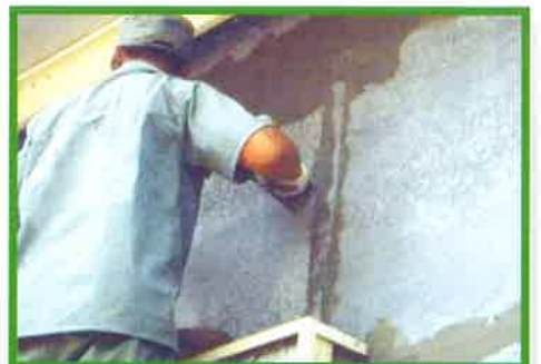
9 Patching up joints with cementitious-based mortar
