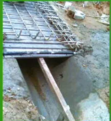
Singapore - ConcritBoard used as Cast-in formwork
