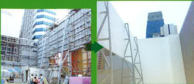
Singapore - Construct New High Wall Above Rooftop
